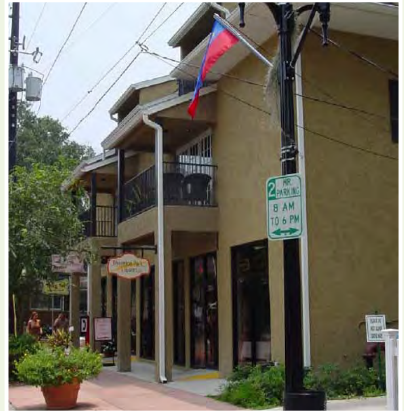
Mixed-Use buildings may incorporate balconies with ground level arcades to serve both upper level residences and lower level businesses.
