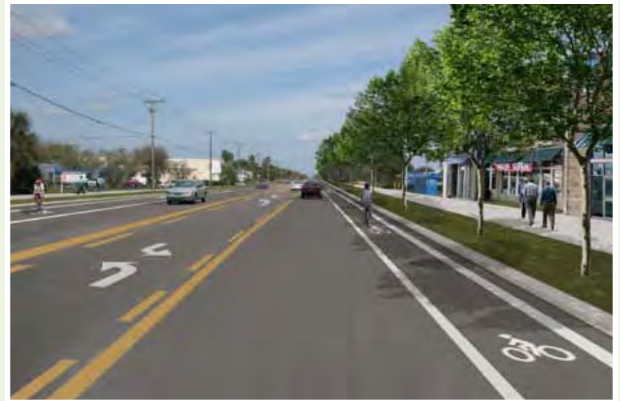
Travel lane widths should be designed to both accommodate expected traffic volumes and balance the needs of other travel modes.
