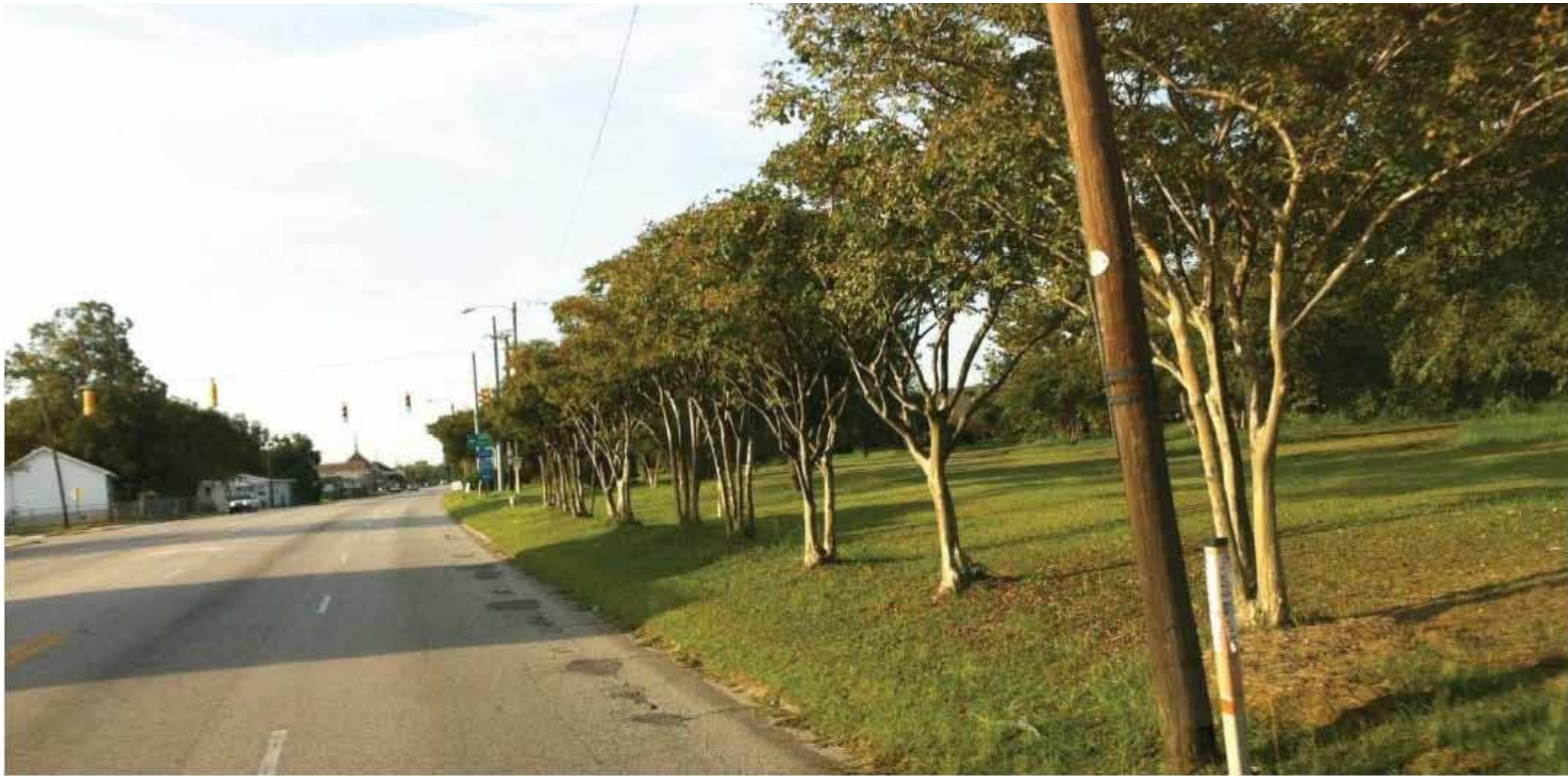
FIGURE B.32 SPRULL AVENUE, EXISTING
