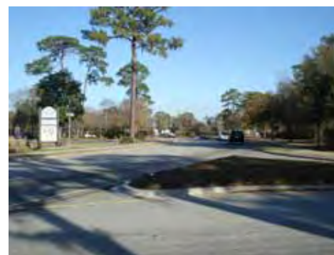
Montague Avenue is one of the main east-west connections in the Neck area.
