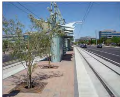
Light Rail Station (Phoenix, AZ)
