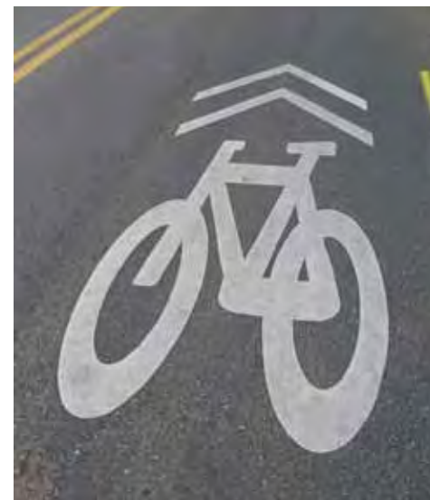
Sharrows show cyclists where to ride and alert motorists of bicycle presence.
