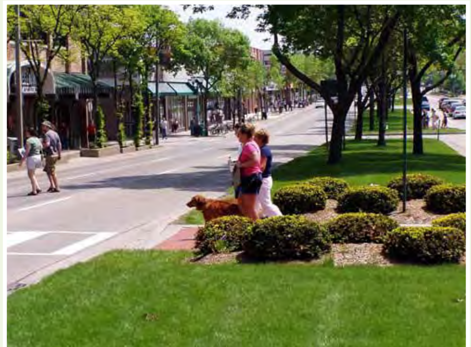
Raised medians help to establish the character of the roadway, provide refuge for pedestrians, and preserve roadway capacity through access management. Images Source: PBIC Library, Dan Burden
