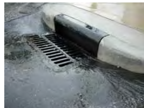
Storm sewers are used to collect surface runoff.
