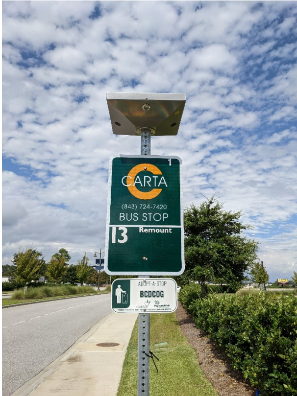
Solar Lighting in Use at CARTA Bus Stop.
