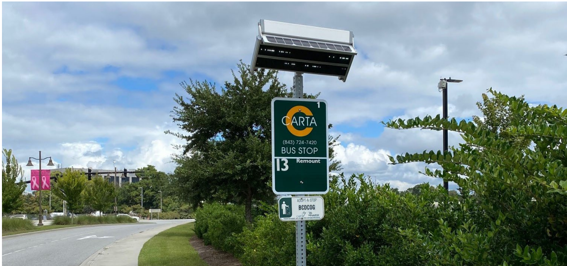
Figure 5-6 Real-Time Arrival Information Board mounted to CARTA Bus Stop
