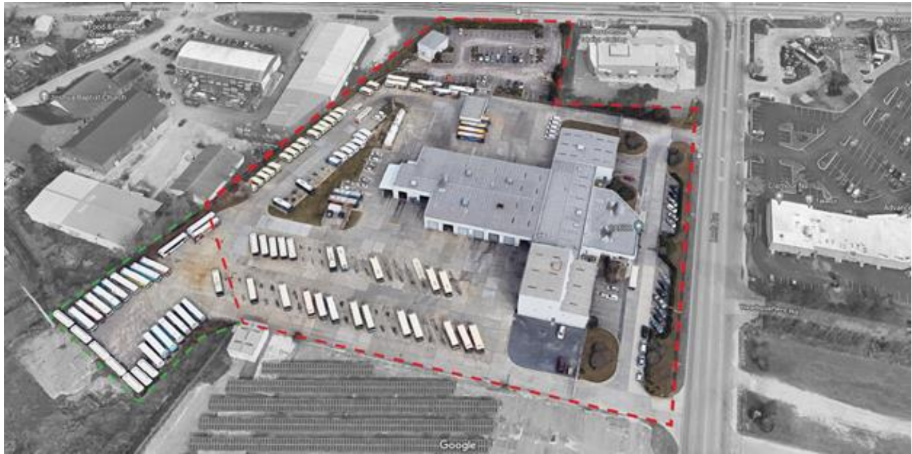
Figure 30: Aerial view of site showing CARTA property bound in red and leased Dominion Energy- property bound in green (source: Google Maps)
