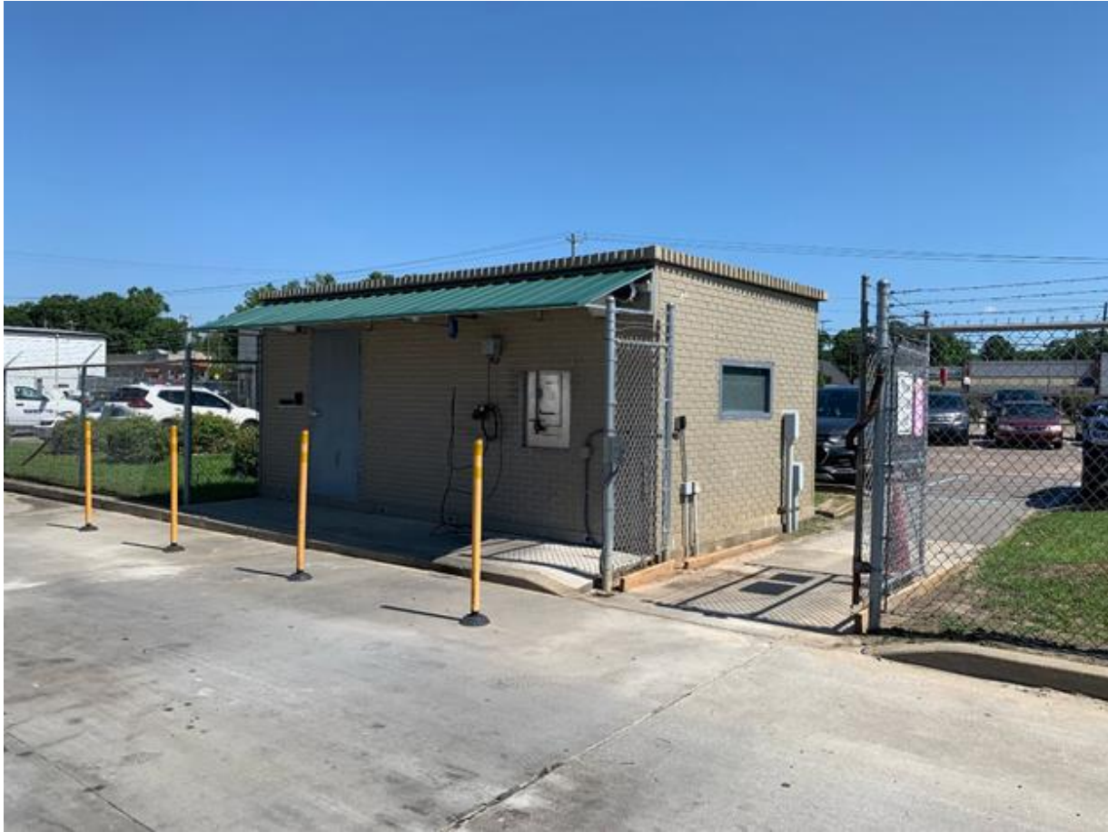
Figure 33: Farebox storage and collection building, with employee parking beyond
