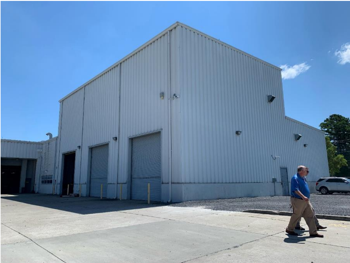
Figure 36: Body shop exterior (3 bays)
