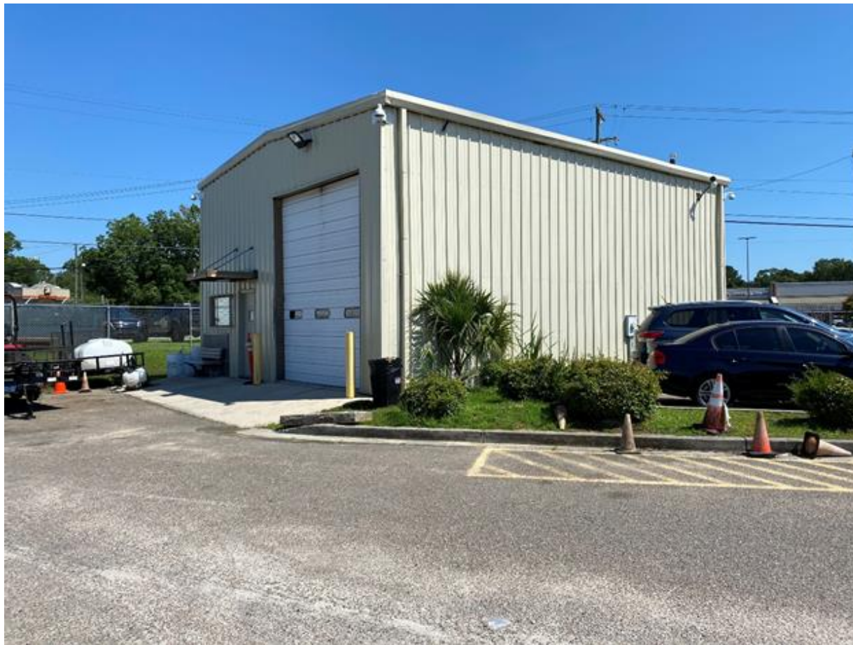
Figure 32: Sign and bus stop maintenance facility
