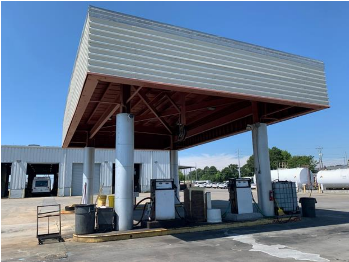
Figure 39: Fueling station and canopy (gasoline and diesel)
