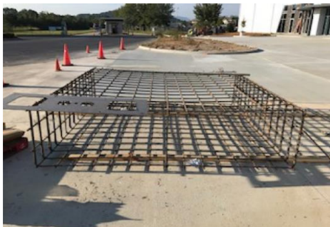
Figure 14: Typical rebar structure for overhead charging pedestal
