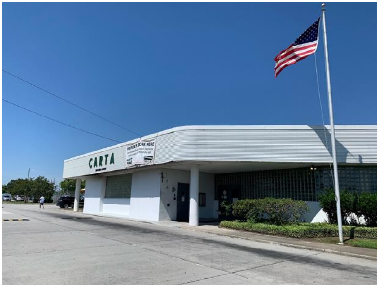
Figure 31: Facility main visitor entry
