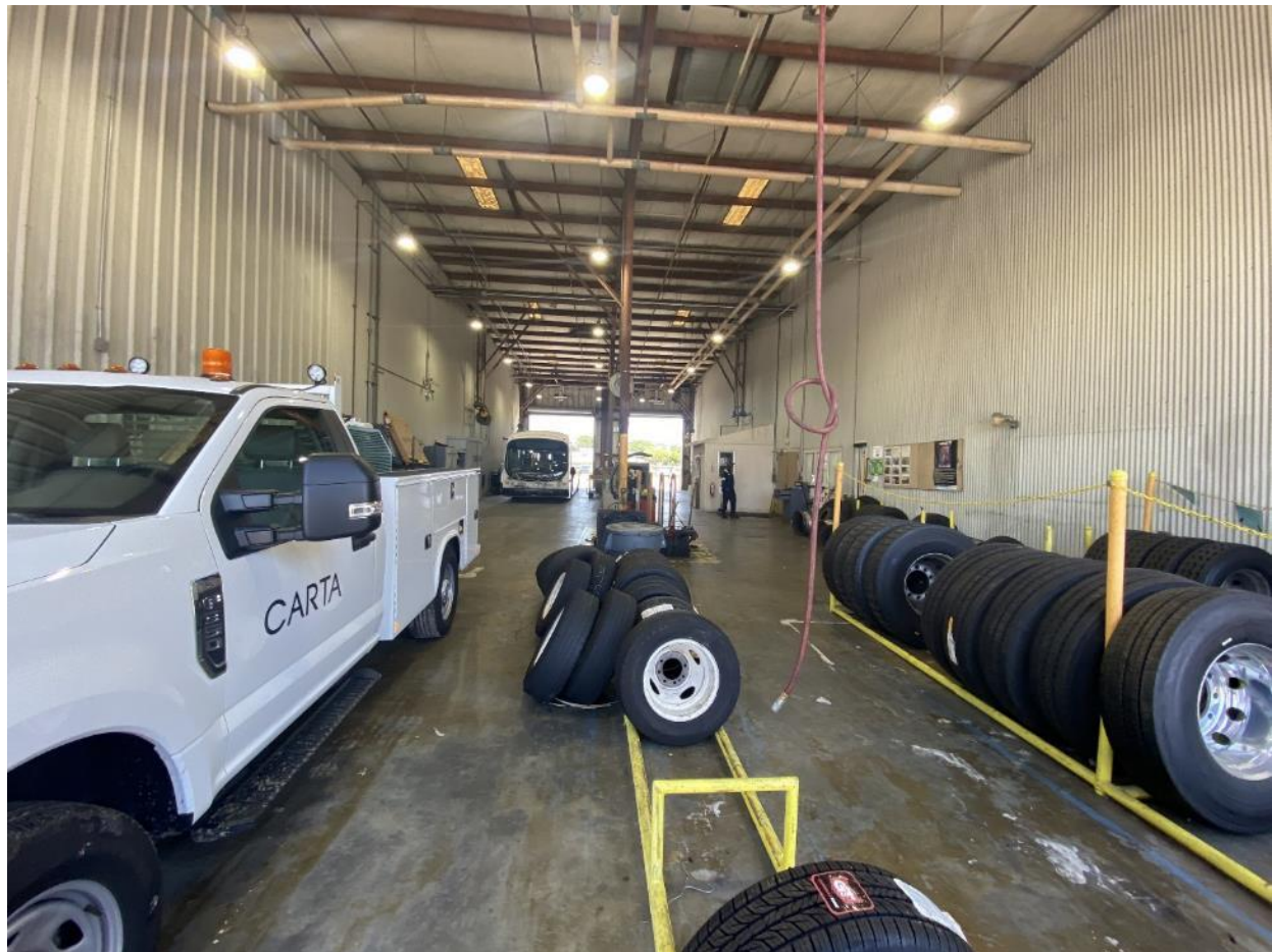
Figure 34: Tire Area and Storage (2 bays in forefront) and Paint Shop (2 bays at far end)
