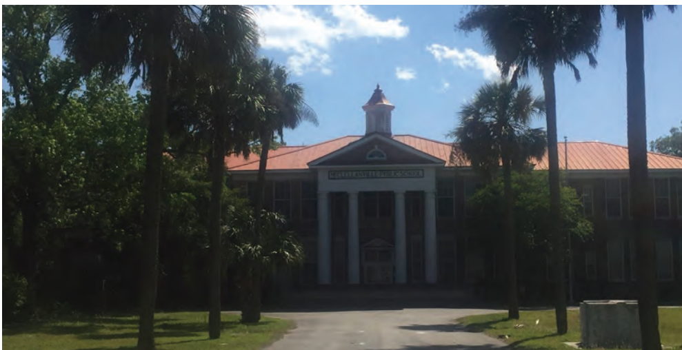
The former and historic McClellanville Middle School has potential to be an adaptive reuse project to house specialized continuing education programs.
