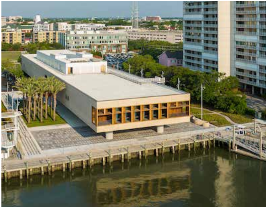
The International African American Museum is set to open in January 2023. (Photo/Ellis Creek Photography)
