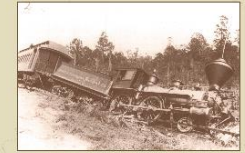
Train derailed from tracks by a four-foot high wall of water when the Charleston earthquake burst the mill dam at Langley Pond near Aiken, SC.
