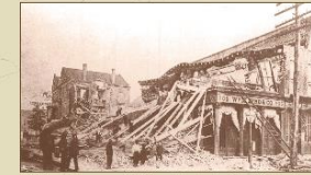
Paint store at the corner of East Bay and Cumberland Streets in downtown Charleston. Damage is result of the 1886 earthquake.
