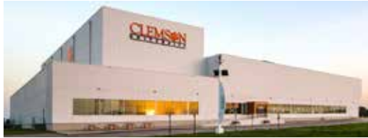
The Clemson University - Dominion Energy Innovation Center in North Charleston. (Photo/Clemson University)
