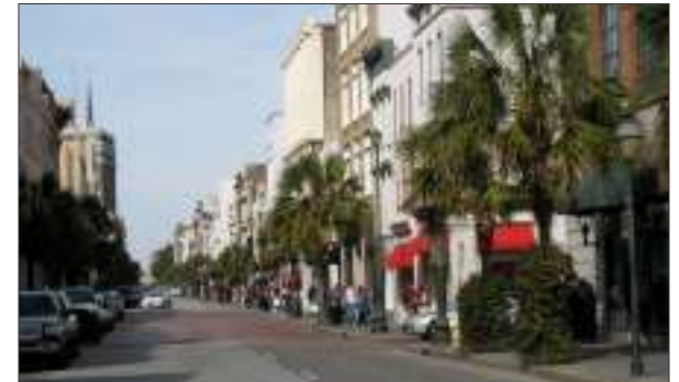
▲ Figure V-1: Home to both urban and rural communities, the Lowcountry is known worldwide for its historic buildings and architecture and walkability. Source: Ron Thomas.
