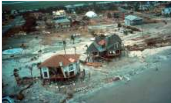
▲ Figure 2-11: Damage from Hurricane Hugo to the barrier islands of Isle of Palms and Sullivan’s Island illustrate the economic and physical destruction from natural hazards in addition to threats to residents’ lives. Source: USGS.
