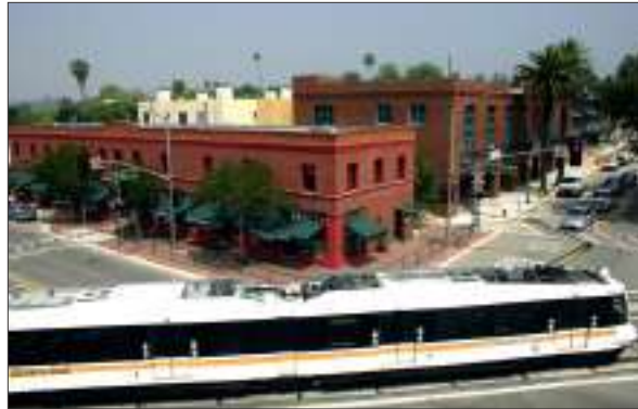
▲ Figure PS-5: The Lowcountry vision of having mixed used development served by transit provides opportunities to maintain the region's historic development patterns, including walkable neighborhoods and town centers.
